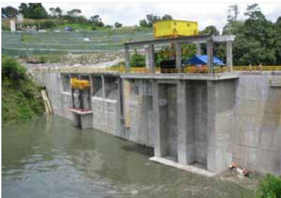
The completed Bajo de Mina Dam produces 36 MW of energy per day.
