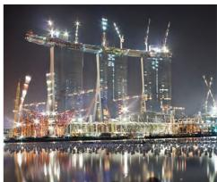
Kryton's KIM-HS was used to waterproof the base slabs, suspended slabs, tunnels, and water tanks.
